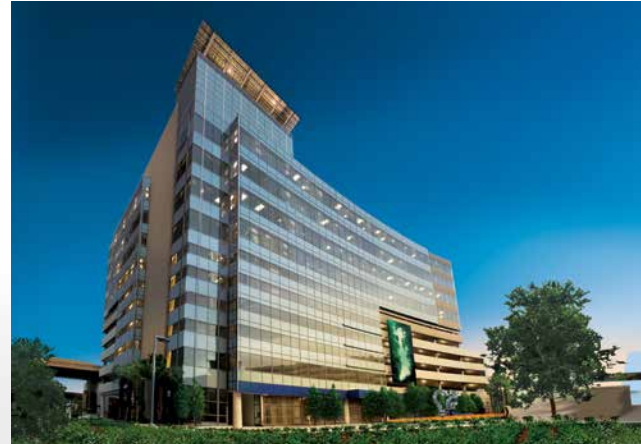
Orlando Utilities Commission
